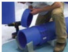
Tack gasket halfway around duct
