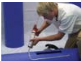
Continuous 1/2" sealant bead.
