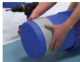
Tack gasket down and apply pressure
