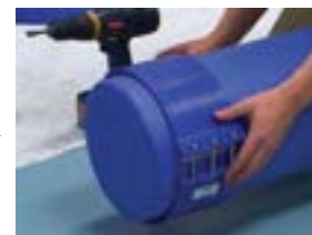
Slide clamp over gasket and tighten screws
