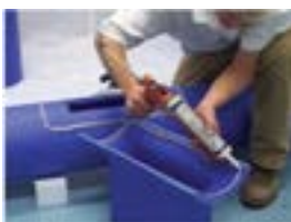
Continuous 1/2" sealant bead.
