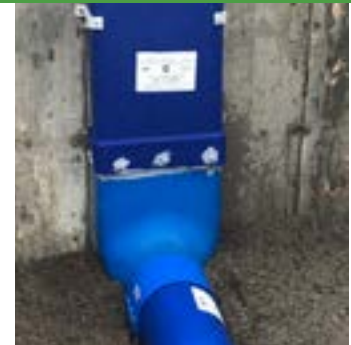
Secure both ends and drill screws into pre-marked locations and cover screw heads with sealant.
