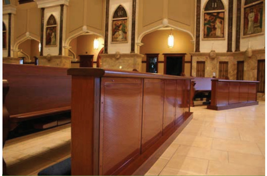
The BlueDuct underground air duct supplies air to the hidden displacement diffusers as indicated by the white arrows.
