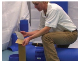
Peel off gasket backing
