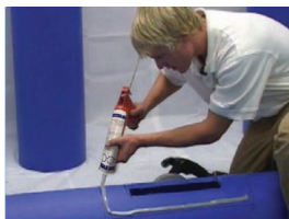
Continuous 1/2" sealant bead.
