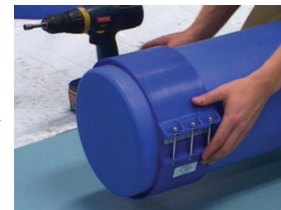
Slide clamp over gasket and tighten screws
