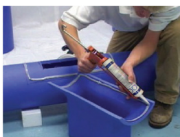
Continuous 1/2" sealant bead.
