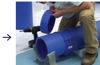
Tack gasket halfway around duct
