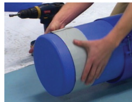
Tack gasket down and apply pressure
