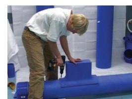
Secure both ends and drill screws into pre-marked locations and cover screw heads with sealant.
