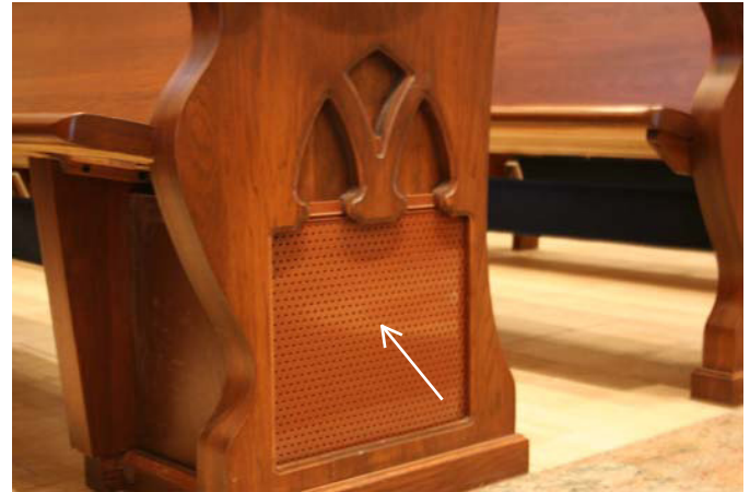
The displacement diffusers are uniquely incorporated into every 3rd pew row as indicated by the white arrows.
