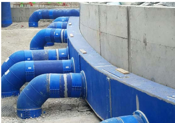
Continus curved radius grill plenum was custom built to fit around the 100ft curved concrete wall shown here.
