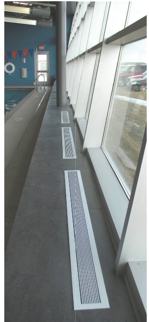
The BlueDuct® underground air duct supplies air to the linear diffusers in the natatorium area
