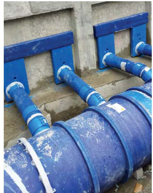
Diffuser boxes were mounted and ducted into the main trunk line after air testing was completed.
